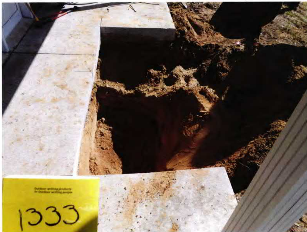
Picture 2: UST 1333Albatross being removed from the excavation.
